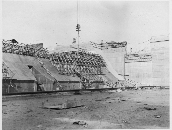
VIEW SHOWING 4 cy. CABLE PLACING DOWNSTREAM FORM ON MONOLITH 17.
