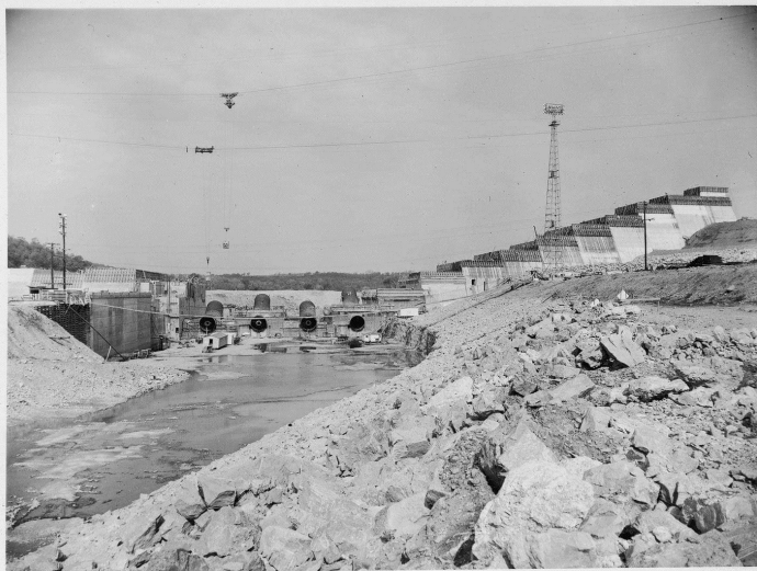
View, looking upstream, showing penstock monoliths and excavated tailrace.
