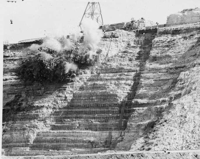
View, looking toward right abutment, showing blasting operation downstream of keyway.
