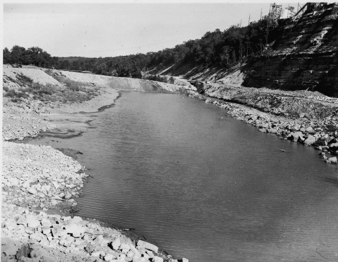
View, looking downstream, showing enclosure of Stage II cofferdam.
