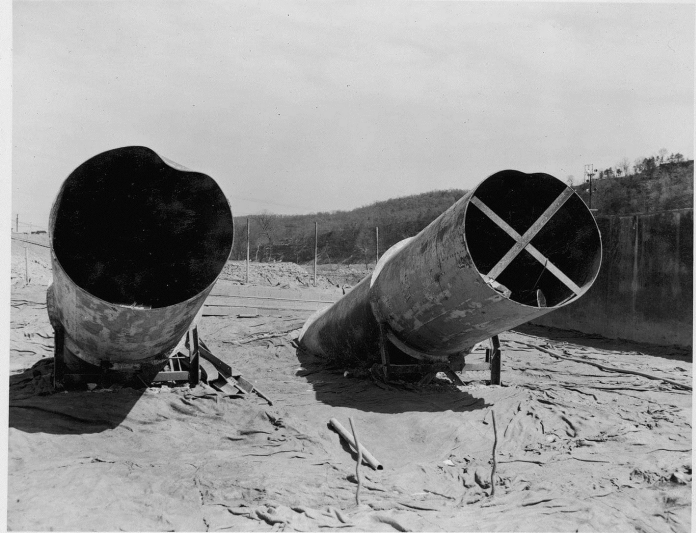
View, looking downstream, showing damaged penstocks.
