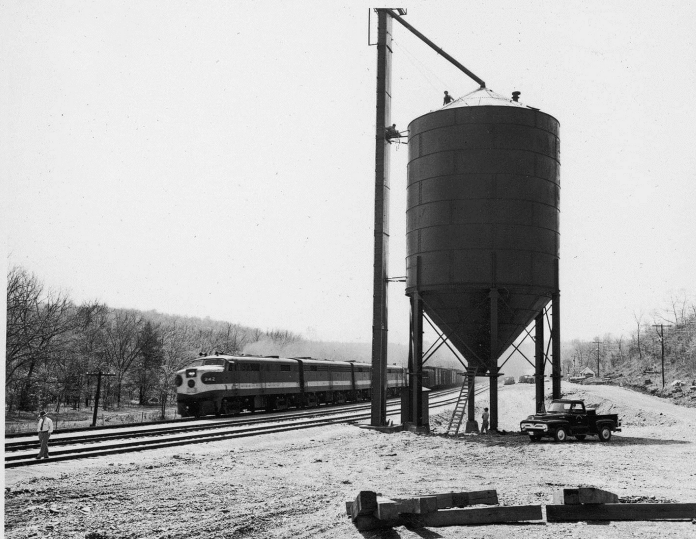
Gretna Siding View of Cement Silo
