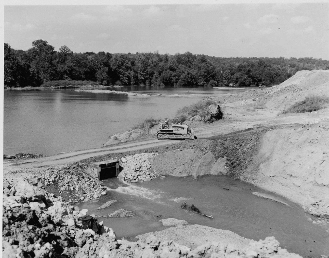
VIEW LOOKING UPSTREAM, SHOWING BOX CULVERT & FILL CROSSING STAGE 2 DIVERSION.
