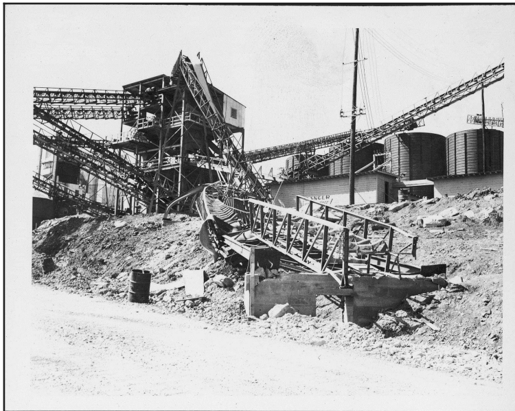
View "F" Conveyor Failure. Looking North from Mid-Point on Up-stream Side.
