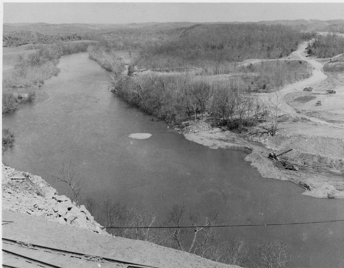
General view, looking upstream from Sta. 63/01, Ra. 6/00. 30 March 1955 Table Rock TR 302
