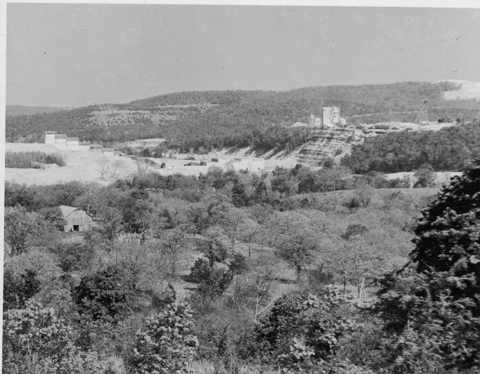
View, looking downstream, showing (L.toR.) earth embankment, concrete section, plant installation & Baird Mountain Quarry.
