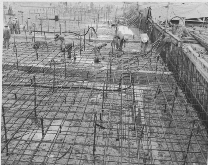
VIEW, LOOKING UPSTREAM, SHOWING SLAB B-3 FOUNDATION IN STILLING BASIN.
