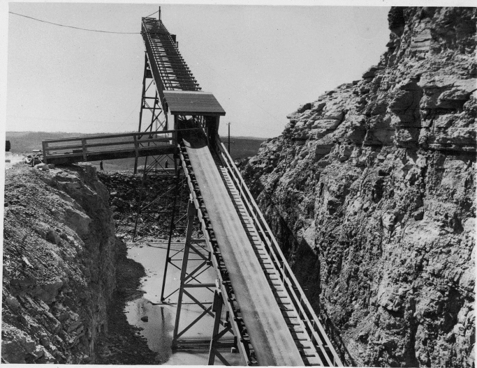
From 42" crusher along 'A' belt to 20,000 ton surge. 23 March 1955
