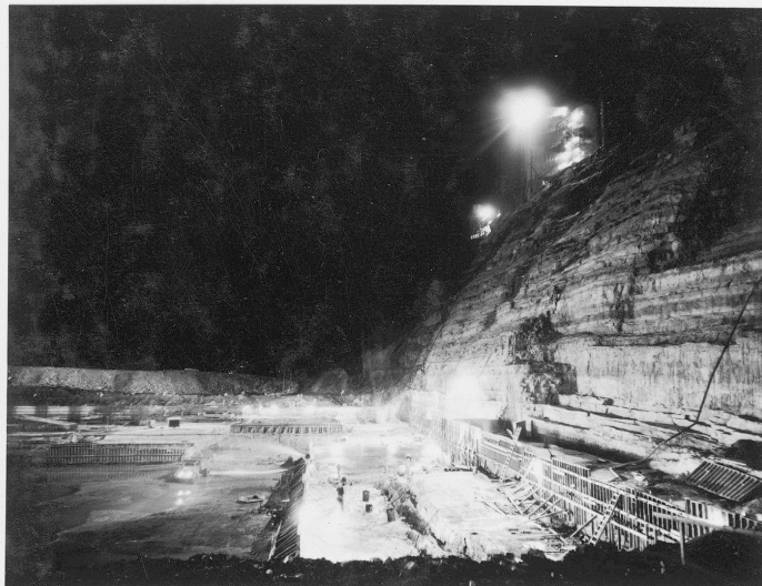
VIEW, LOOKING DOWNSTREAM, SHOWING NIGHT OPERATIONS IN MONOLITH 24.
