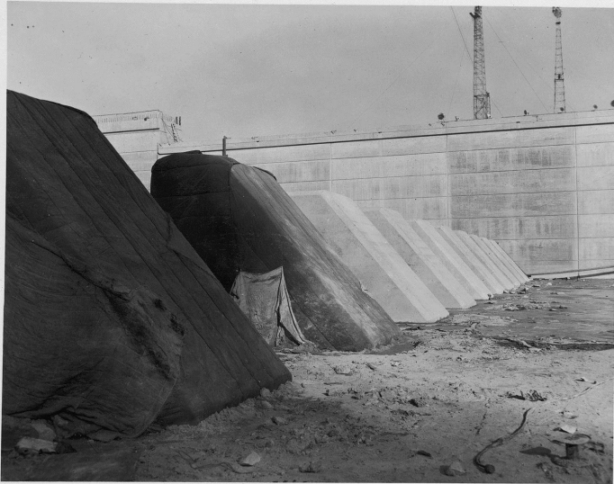
VIEW SHOWING COLD WEATHER PROTECTION ON BAFFLES IN STILLING BASIN.
