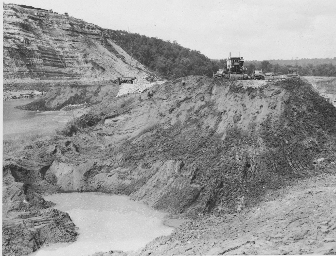
View, looking upstream, showing excavation of Stage 1 cofferdam partly completed.
