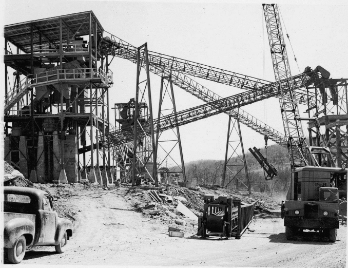
View installation of conveyors at transfer station, looking downstream right abutment; on left is the screening plant.
