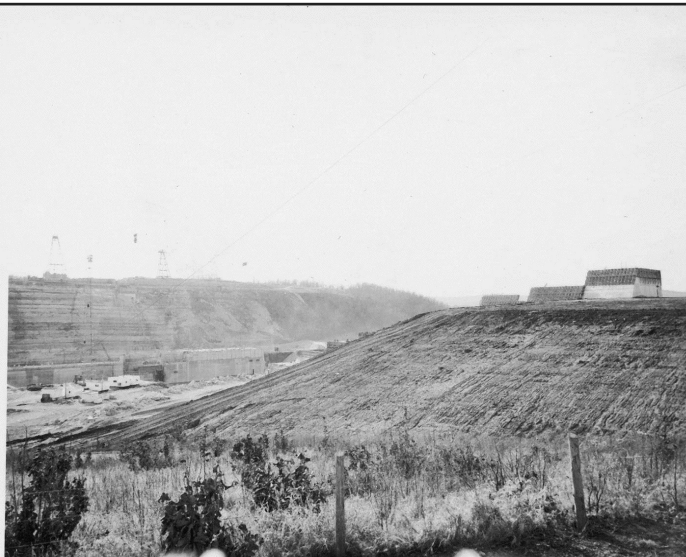
VIEW LOOKING TOWARD RT. ABUTMENT FROM THE OVERLOOK.
