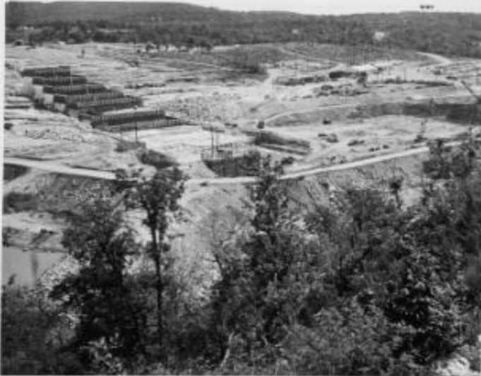
View, looking east, showing progress on left abutment.
