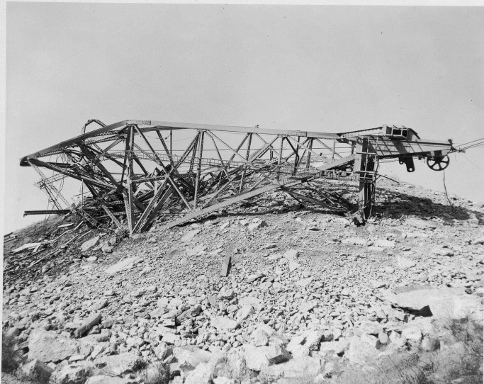
View, looking upstream, showing collapsed 8 cy. tail tower.
