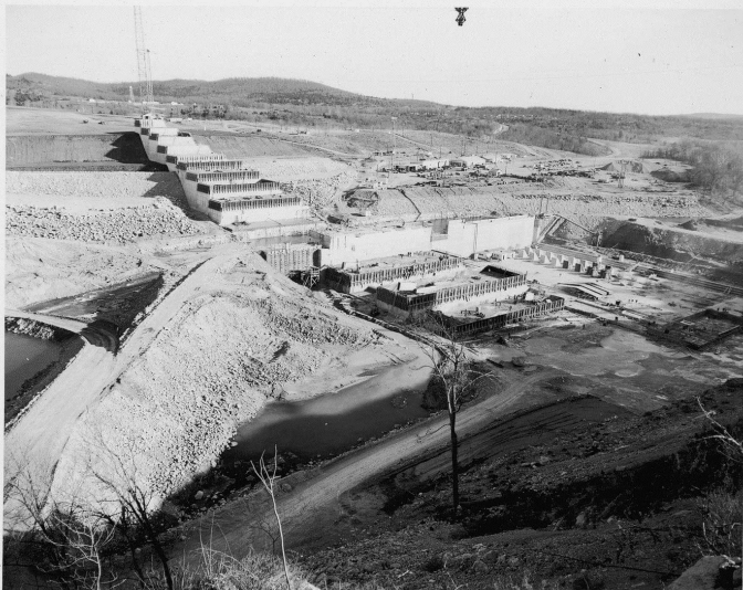
VIEW LOOKING NORTHEAST AND DOWNSTREAM FROM STA. 63+00, R7+00.
