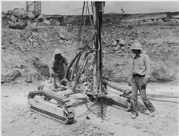
Line drilling close-up at Sta. 48+00.
