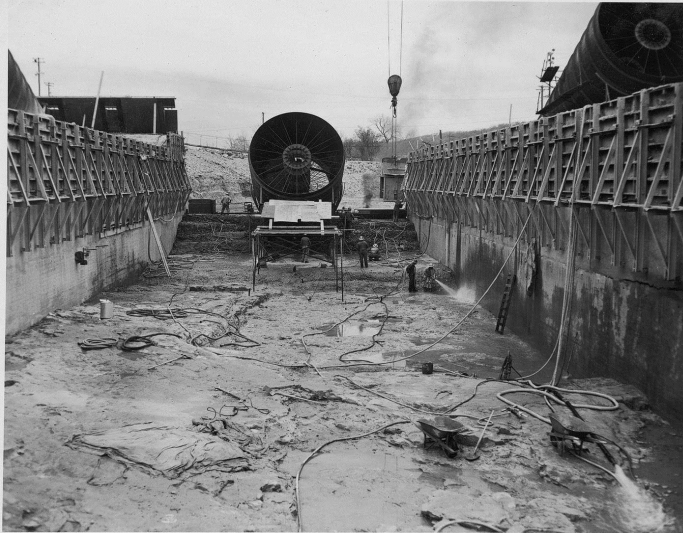
View, looking downstream, showing Monolith 12 foundation.
