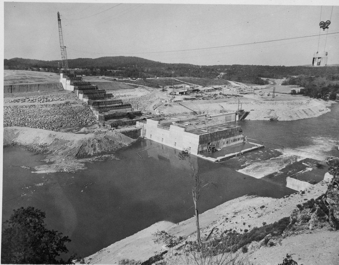
View looking northeast and downstream from Station 63+00, Range 7+00.
