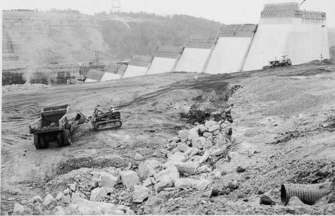
VIEW LOOKING UPSTREAM, SHOWING REMOVAL OF ROCK ON DOWNSTREAM WRAPAROUND SECTION.
