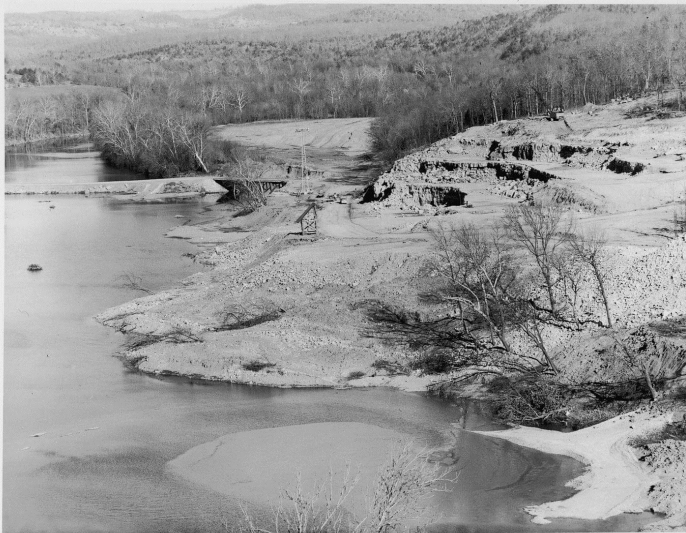
VIEW, LOOKING UPSTREAM, SHOWING ROCK FILL QUARRY.
