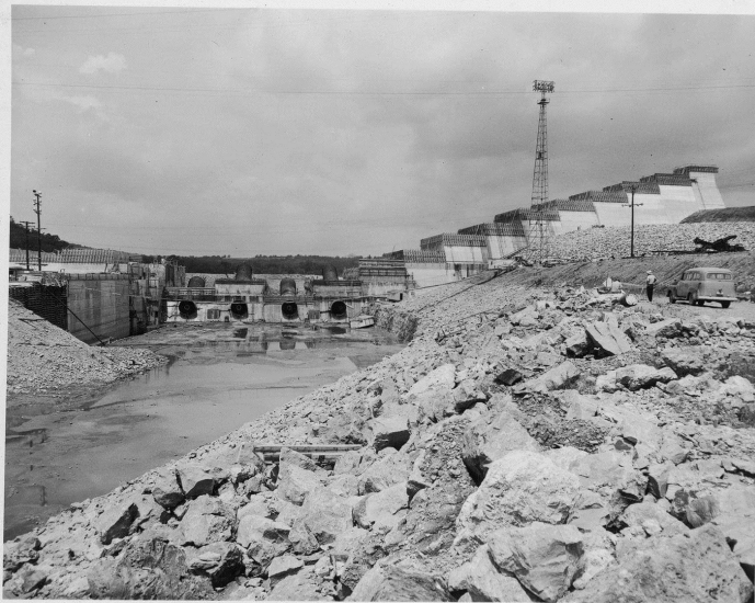
View, looking upstream, showing penstock monoliths and excavated tailrace.
