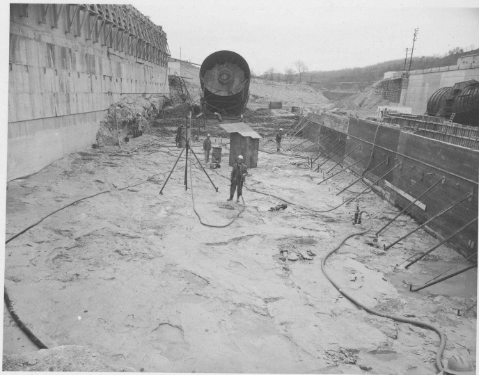
View, looking downstream, showing Monolith 11 foundation.
