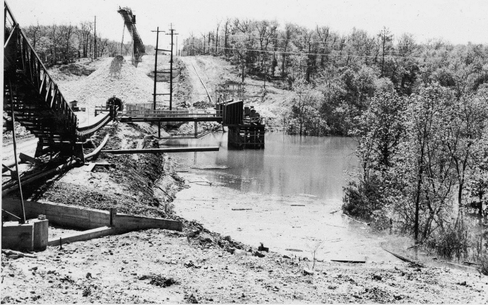
VIEW SHOWING 40,000 TON SURGE PILE, UPSTREAM SETTLING POND, AND PUMP STATION.
